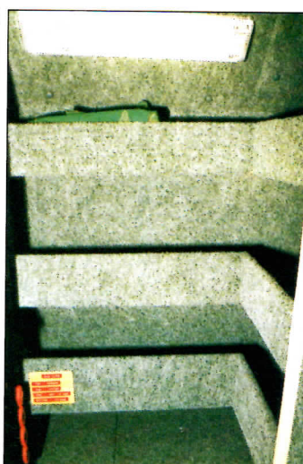
Here's how to make use of wardrobe space. The hanging area remains the same, but Bill has taken account of the sloping walls to add extra shelves. The finishing touch – interior illumination when the door opens.
